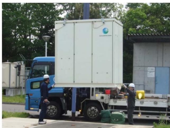
Fig. 3 2 kW turbo refrigerator component
