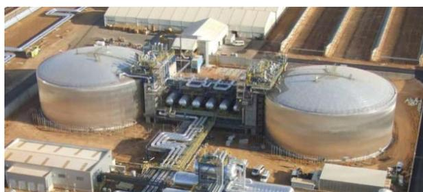
Fig. 1 23m-diameter tank can store the equivalent of 300 MWh energy
