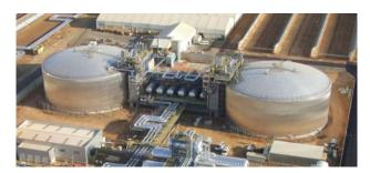
Fig. 1 23m-diamter tank can store the equivalent of 300 MWh energy
