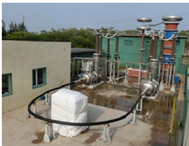
Fig. 2 Preparation of the short circuit simulation test at Shenyang Furukawa Cable
